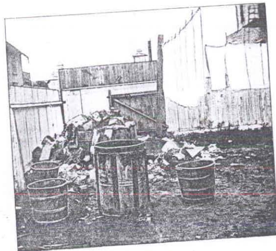
A Neglected Back Yard.
