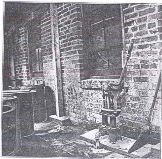
Well in Polluted Ground Beneath Building.
