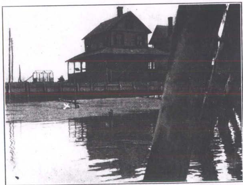
Sewer discharging near clam grounds, Highland Beach. (Page 184.)
