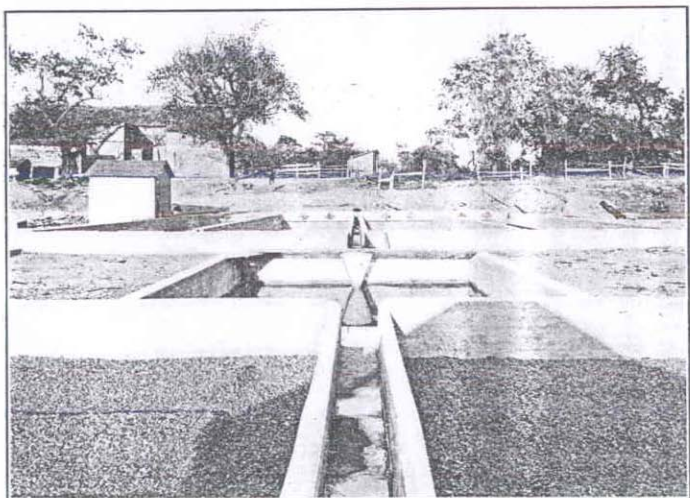
Millville. View Showing Aeration Well.
