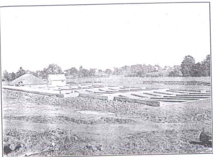
Collingswood. Septic Tank and Contact Beds.
