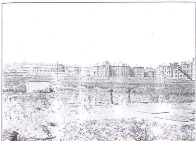
Overbrook. Septic Tank.
