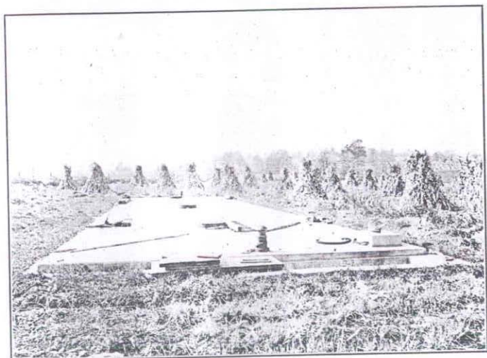
Princeton. North-east Field. Septic Tank.
