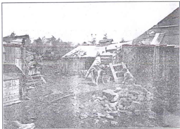
View showing unsanitary conditions surrounding a dairy in which 46 cows are kept and about 400 qts. of milk produced daily.
