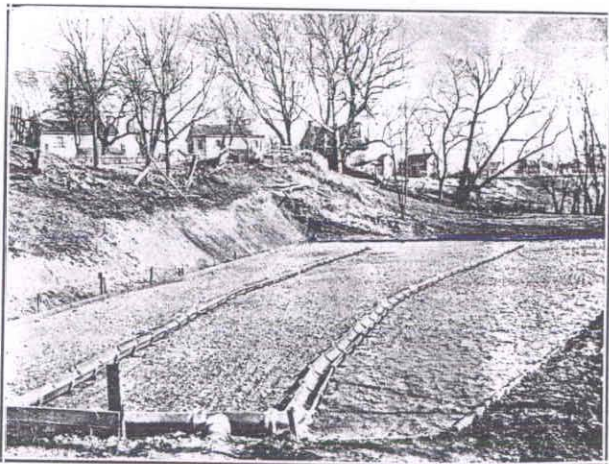
WOODSTOWN: New Sand Bed for Town Plant.
