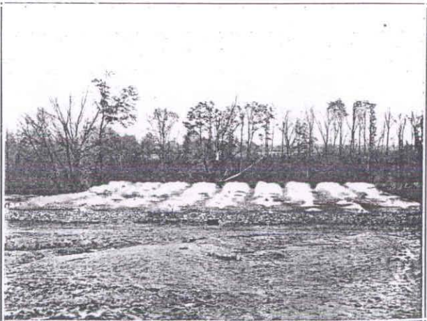
HADDONFIELD: Sprinkling Filter in Action.
