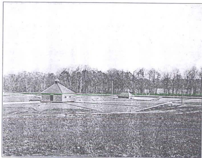
MORRISTOWN: Sewage Disposal Plant.
