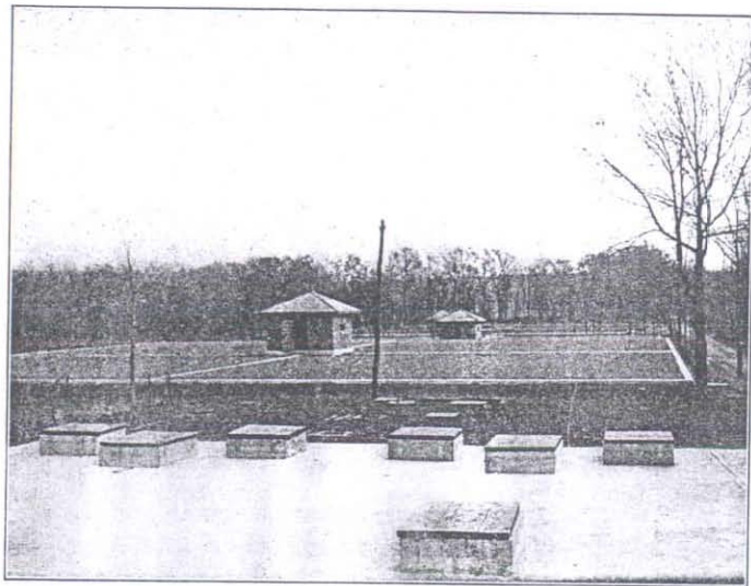
CHATHAM-MADISON: Sewage Disposal Plant.
