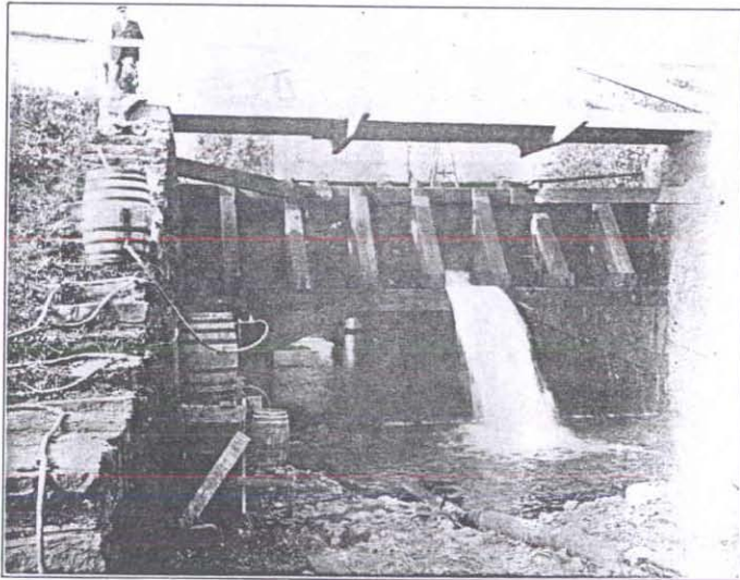
LAMBERTVILLE: State Emergency Hypochlorite Plant in Use.
