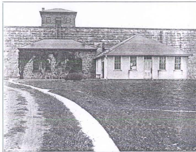
BOONTON: Hypochlorite House for Jersey City Supply.
