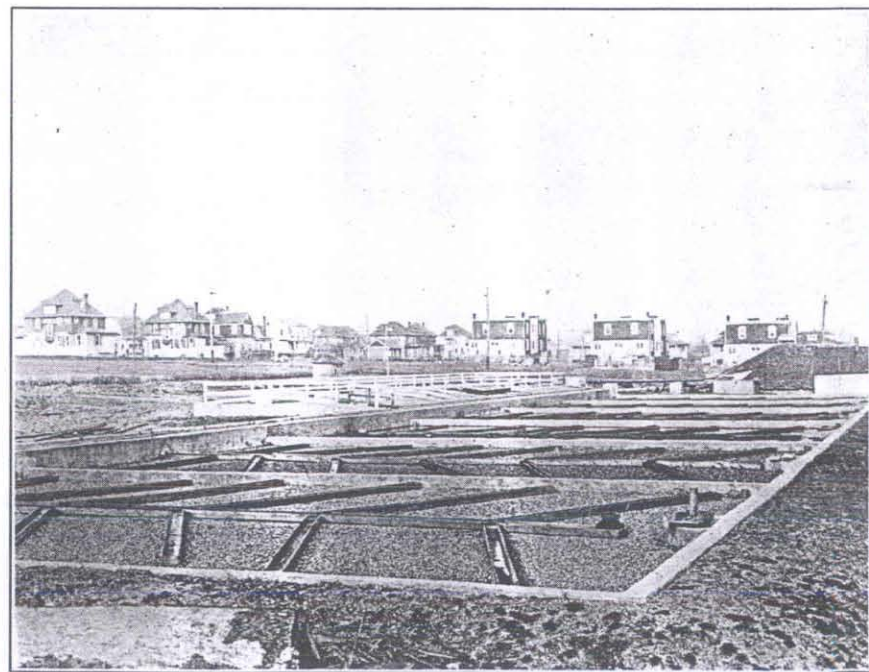
COLLINGSWOOD: Sewage Disposal Plant.
