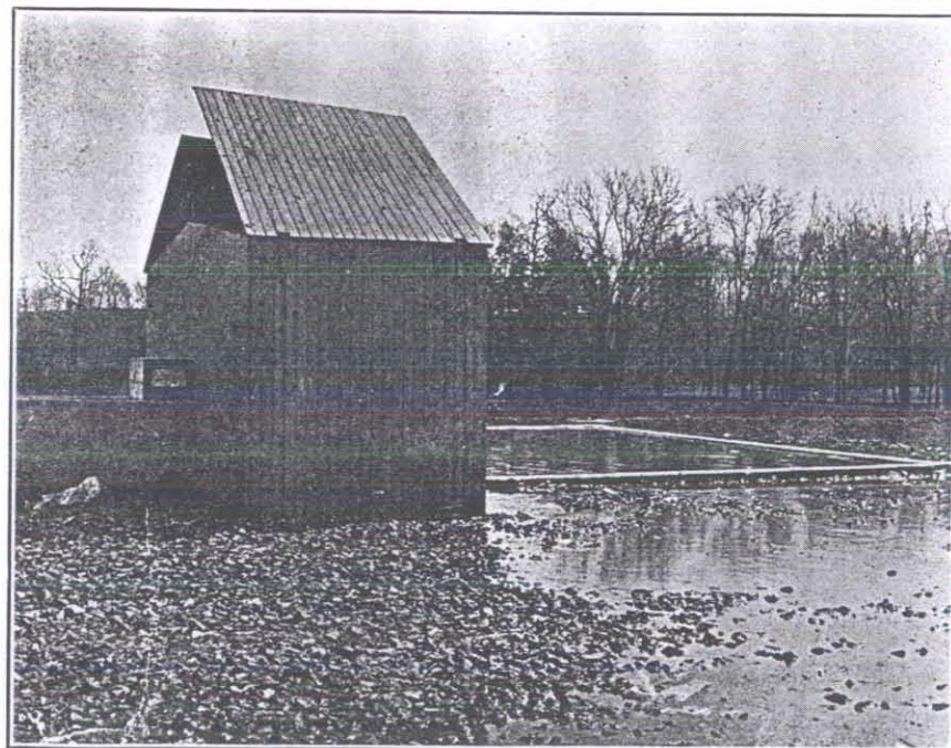
SKILLMAN: Sewage Disposal Plant, Beds Flooded.
